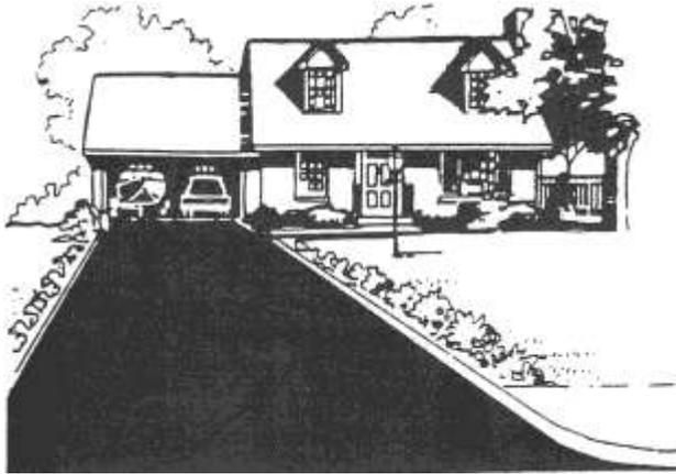
Asphalt concrete pavement is a popular choice for residential driveways. Properly designed and constructed, it stays smooth, sound and attractive in appearance over many years. Flexibility allows the pavement to conform to minor subgrade settlements and still retain a continuous surface free of abrupt bumps.
